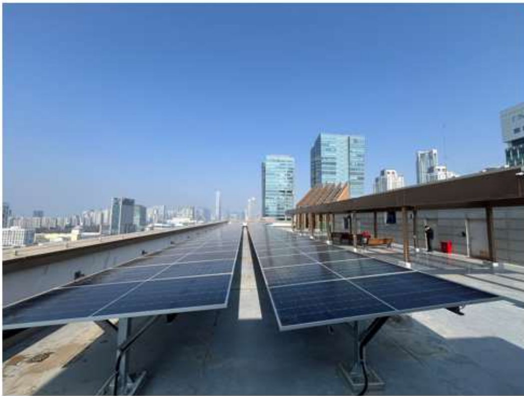
Solar panel installation
