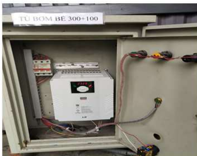
MCNEX VINA Inverter Installation
